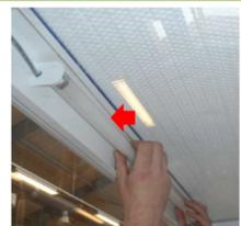
4. The fluorescent tubes are mounted in rotating sockets. Rotate the tube carefully into the removal position, and then remove it from the socket. Insert the new tube and rotate it into the working position.
